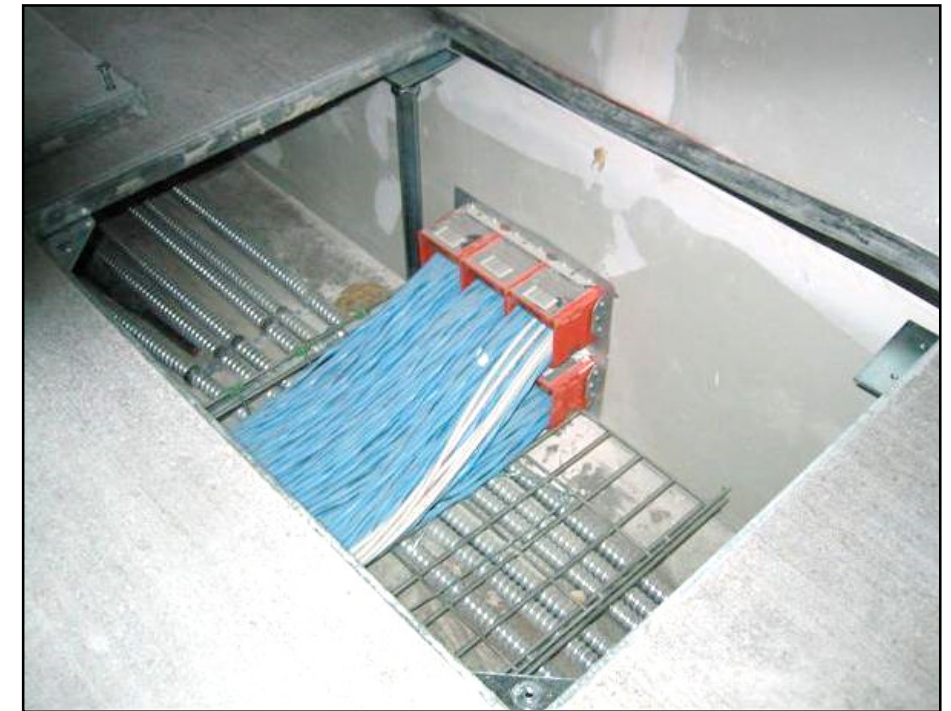
Below raised floor
