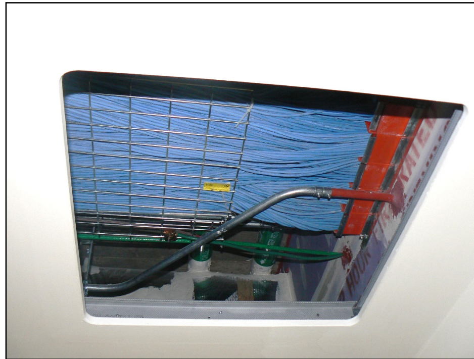
Above the ceiling
