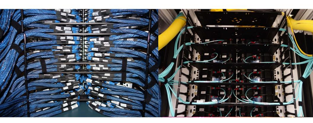
Added recommendation to consider needs for proper labeling, cable routing, cable management, and ability to insert and remove cords without disrupting existing or adjacent connections when selecting patch panels.
