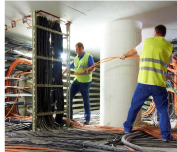
Fiber cuts /High loss
