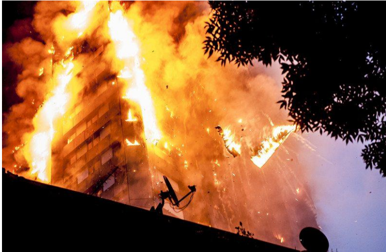
Fire rapidly engulfed Grenfell Tower in London Guilhem Baker/LNP/Rex/Shutterstock
